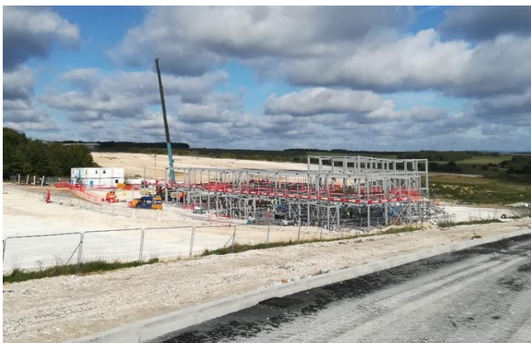
St. Michael's School build progress, Larkhill.
